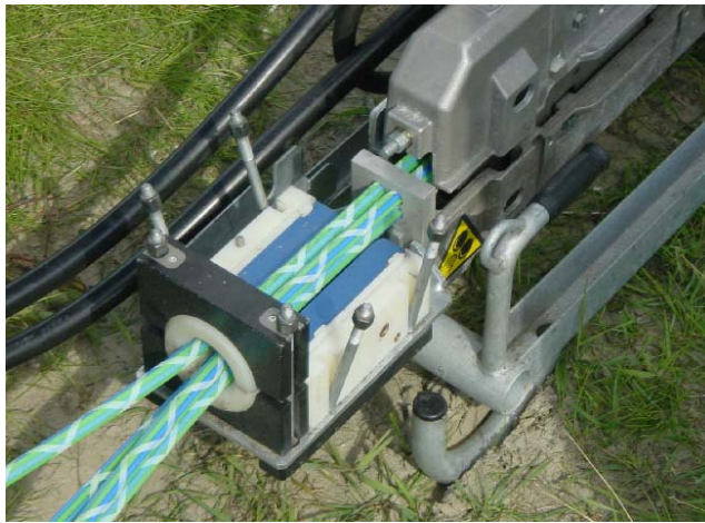
Figure 5 Jetting 4 sub-bundles, each 6 \mu ducts of 4 mm around strength member, for FttH
